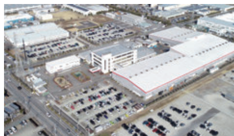
● Kofu Plant 甲府工場 Site: 38,292 m 2 (412,172 sq.ft.) / Floor space: 25,957 m 2 (279,399 sq.ft.)
