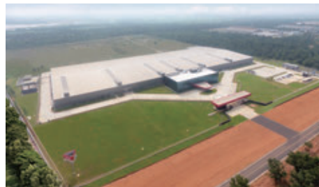
●THK India Pvt. Ltd., Headquarters and Sri City plant (India) Site: 205,094 m 2 (2,207,620 sq.ft.) / Floor space: 36,691 m 2 (394,938 sq.ft.)
