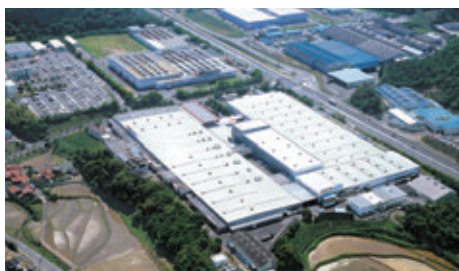
● Yamaguchi Plant 山口工場 Site: 160,798 m 2 (1,730,818 sq.ft.) / Floor space: 77,912 m 2 (838,641 sq.ft.)
